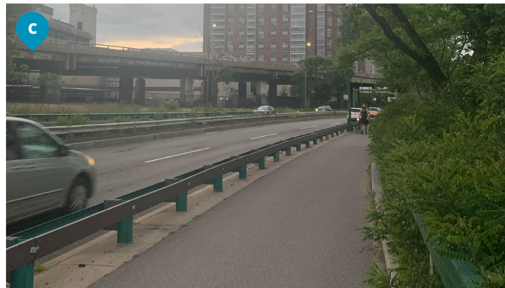
PDW Path Adjacent to SFR Narrow path (no separation of peds and cyclists) with inadequate buffer from the road
